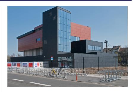
Construction of a signalling centre for the Belgian railways and demolition of an existing post office building. The complete building forms a Faraday cage to protect the railway signalling. This was accomplished by earthing 4,100 m² of concrete walls and interconnecting all concrete reinforcement.
