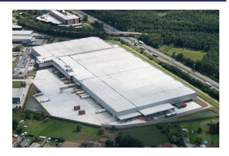
On a site of just over 10 hectares along the E313 motorway, we built a 50,000 m<sup>2</sup> distribution centre with 62 loading docks. From this location, CASA shops have been supplied throughout Europe since 2017. Thanks to a space that can accommodate 65,000 pallets, the company can save 5,000 freight trips a year. In addition to the warehouse and the necessary technical areas, the new building comprises 5,000 m<sup>2</sup> of offices spread over four floors.
