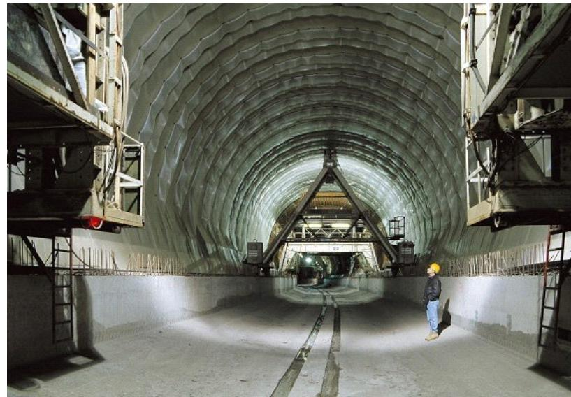
Double 1,300 m tunnel, each tunnel with road interchanges at entrance and exit. The tunnels run 50 m below the ground, mostly under a built-up zone. The shoring consists of 30 cm of shotcrete and passive bolting with 1.5 metre intervals.
