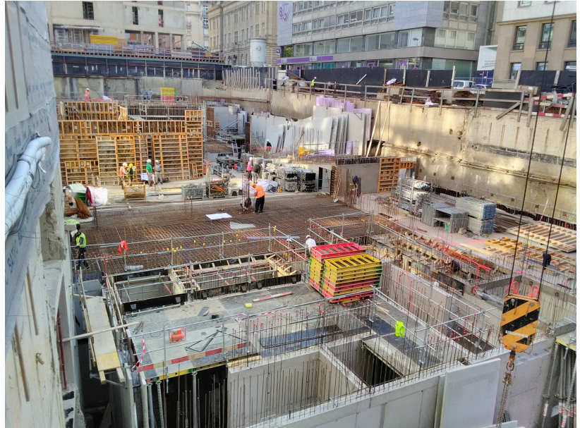
Construction of a residential building.
