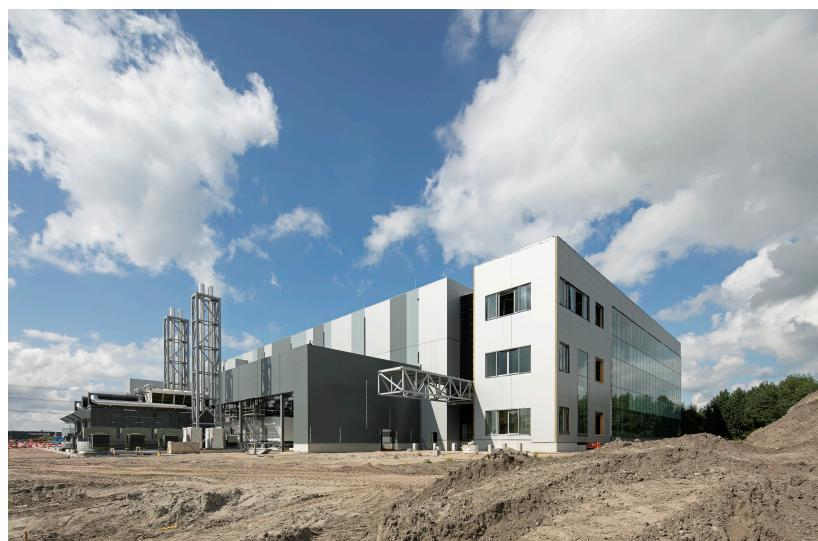
Realisation of the closed shell of the new campus for US data centre operator CyrusOne with a capacity of 72 megawatts. The structure consists of 3,500 tonnes of steel and 4,000 m<sup>3</sup> of concrete and is founded on 3,500 foundation piles.
