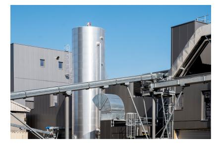
Since 1875, this malting plant has been processing grain, barley and wheat into typical malt that is used in special beers such as Westmalle, Westvleteren, Rochefort, Duvel, but also in baking. In Stabroek, we helped build the drastic expansion of the malting plant. The work specifically required particularly technically sophisticated expertise. The concrete walls of the sprout boxes (9 by 9.5 metres), for instance, could only show a deviation of maximum 1.5 mm.
