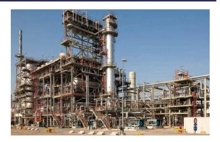
This project was part of a worldwide effort to expand and modify three refineries in Europe (including Antwerp) and the US to produce cleaner diesel. This increased the production of low sulfur diesel in these plants by over 22 million litres per day. The High Pressure Hydrotreater is a system that desulfurises diesel with hydrogen under high pressure.
