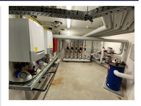
HVAC and SANITARY Renovation of listed building Heat production gas-fired boilers Cold production with monoblock chiller Ventiloconvectors 2 Air handling units for cooling and heating with electric steam humidifier and dehumidification.
