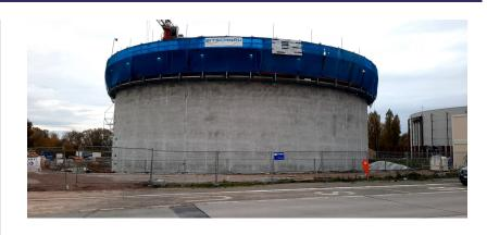
Construction of a cylindrical concrete drinking water reservoir with an inner diameter of 38.4 m, a wall (via sliding formwork) with a thickness of 45 cm and a height of 16.5 m, including surrounding construction.
