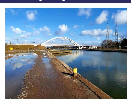
This 600 tonne steel arch bridge is 74 metres long and over 17 metres wide, and is expected to improve access and road safety in and around the business park adjacent to the Brussels-Charleroi Canal. The bridge was built in the workshop in twelve transportable sections. The individual sections were then assembled on site along the canal and finally transported by ship to their final position with the necessary care and precision before being placed.
