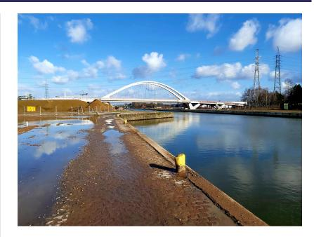
This 600 tonne steel arch bridge is 74 metres long and over 17 metres wide, and is expected to improve access and road safety in and around the business park adjacent to the Brussels-Charleroi Canal. The bridge was built in the workshop in twelve transportable sections. The individual sections were then assembled on site along the canal and finally transported by ship to their final position with the necessary care and precision before being placed.
