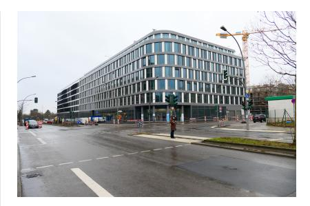
Design and build of two buildings with eight floors and 25,000 m<sup>2</sup> of office and retail space. The project also has a 9,000 m<sup>2</sup> underground car park. This project will be LEED Gold-certified when completed. LEED stands for 'Leadership in Energy and Environmental Design' and assesses construction projects in terms of sustainability in the broadest sense of the word.
