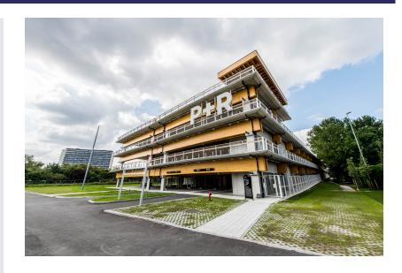
This ultramodern 'park and ride' car park (12,000 m²) in Merksem has room for 690 cars and 150 bicycles and 18 charging points for electric vehicles. The building is characterised by its light and open construction, in which wooden beams play the main role.
