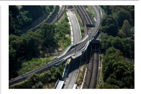
The project consisted of infrastructure work along the track bed platform where railway lines L124 and L26 intersect. Several bridge decks were renovated and noise barriers installed, including 2,000 m² of green walls. For the Moensberg station at Uccle, new platforms have been built. Simultaneous with these main works diverse road, bedding, demolition, earth- and sewerage works were performed.
