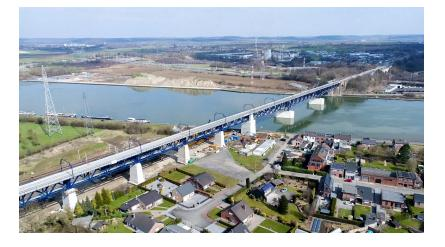
The 523 meter long Pont des Allemands, in use since 1917, is one of the most remarkable works of art on the Belgian railway network. Every day, about 80 freight trains use it to cross the Meuse. A century after its construction, the viaduct was due for a rejuvenation. As part of a complete renovation of this viaduct, we installed a new bridge deck, among other things. The tracks and overhead lines were also renewed and the eight concrete piers were reinforced.
