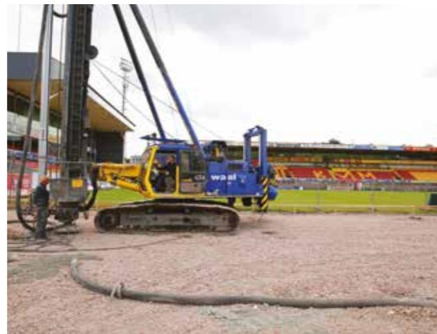
There is increasing demand to build on less stable soil. Pile foundations are the solution for this. They transfer the forces to the deeper layers, capable of bearing the load. *The DE WAAL group specialises in soil displacement systems and can install both driven and vibration-free systems, including in existing buildings.*
