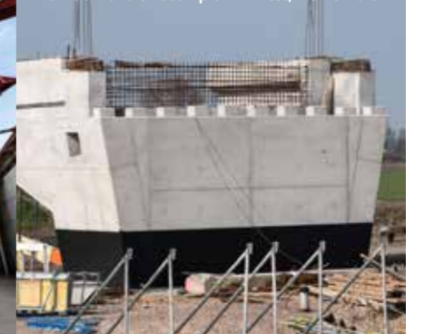
Traffic on- and exit complex R4-West, Rieme-North
